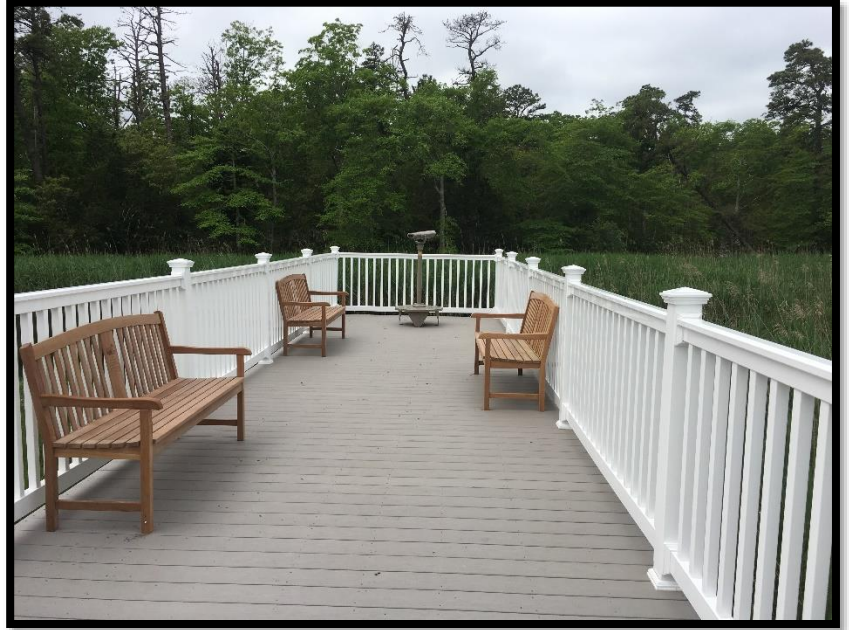
Figure 8. Boardwalk and observation platform along the LOE at the Grassle Marsh Trail
